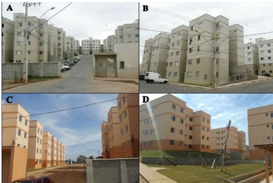
Figura 10 - Residencial “Alfenas” (2013) e Residencial “Jd. São Carlos” (2015).
